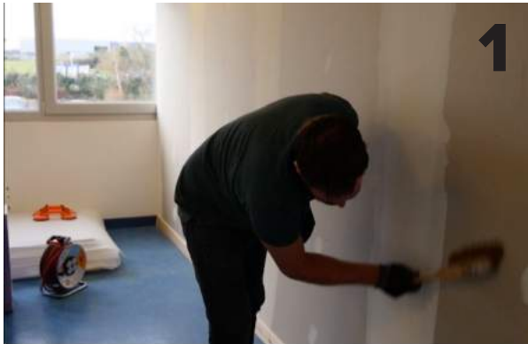
CLEAN THE WALL BEFORE INSTALLATION
