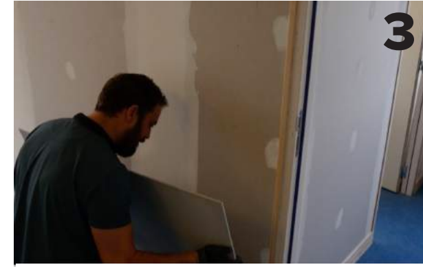
FIT THE SLIMBETON® STARTING FROM BOTTOM TO TOP
